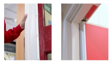
For new builds and refurbishments efforts should be made to completely avoid, by design, any pinch points presented by doors and gates, before consideration is given to guarding or other precautionary measures.
