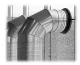
Local exhaust ventilation is primarily provided to help meet the requirements of the Control of Substances Hazardous to Health Regulations. People can develop lung diseases such as occupational asthma because they breathe in too much dust, fume, vapour and mist or other airborne contaminants.
