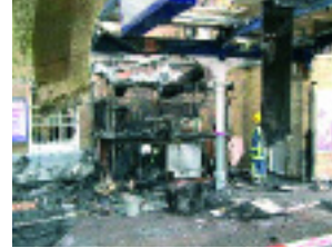
Figure 6: Fire in a retail unit on a platform (arson) (courtesy of Network Rail)
