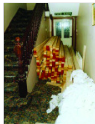
Figure 9: A blocked corridor with incorrect signage
