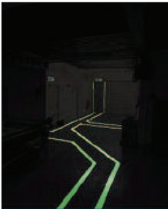
Figure 53: A 'way-guidance' system
